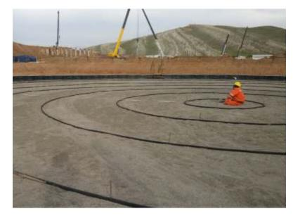
Tubular anodes are supplied with the specified cable connected to anode mid-length by in-house developed internal connection to minimise anode to cable resistance and not to lower anode surface area.
